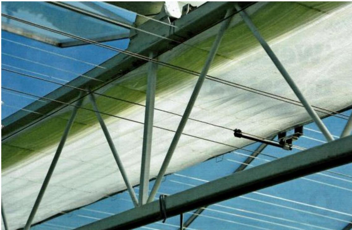
The upper screen fabric is pressed neatly against the upper truss when closed. The lower screen fabric makes use of a lowered drag profile, so that it is pulled under the truss when
