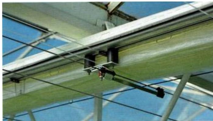
In addition, the extra upper screen sagged somewhat between the suspension points, which did not result in a nice even cavity thickness. An alternative, with a fully double wire bed, would have made the costs considerably higher, which was undesirable.
